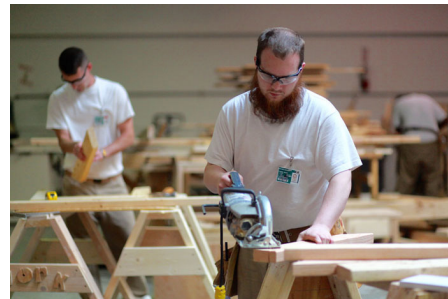
Incarcerated students learn valuable skills that put them on a path to find a well-paying job upon release. This student is working as part of the Construction Trades Apprenticeship Program. Photo courtesy of the Department of Corrections.
